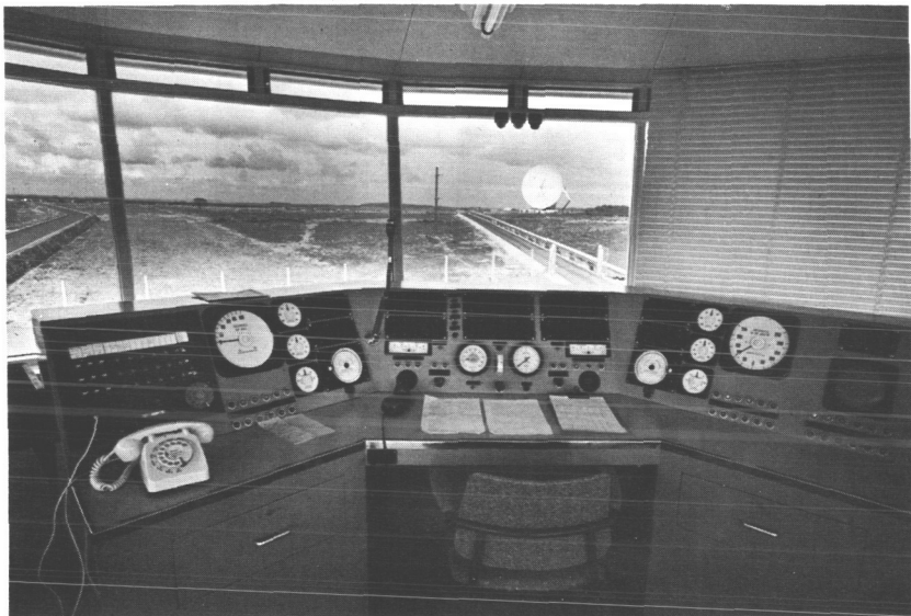
Fig. 8 — The aerial steering position in the control tower.
