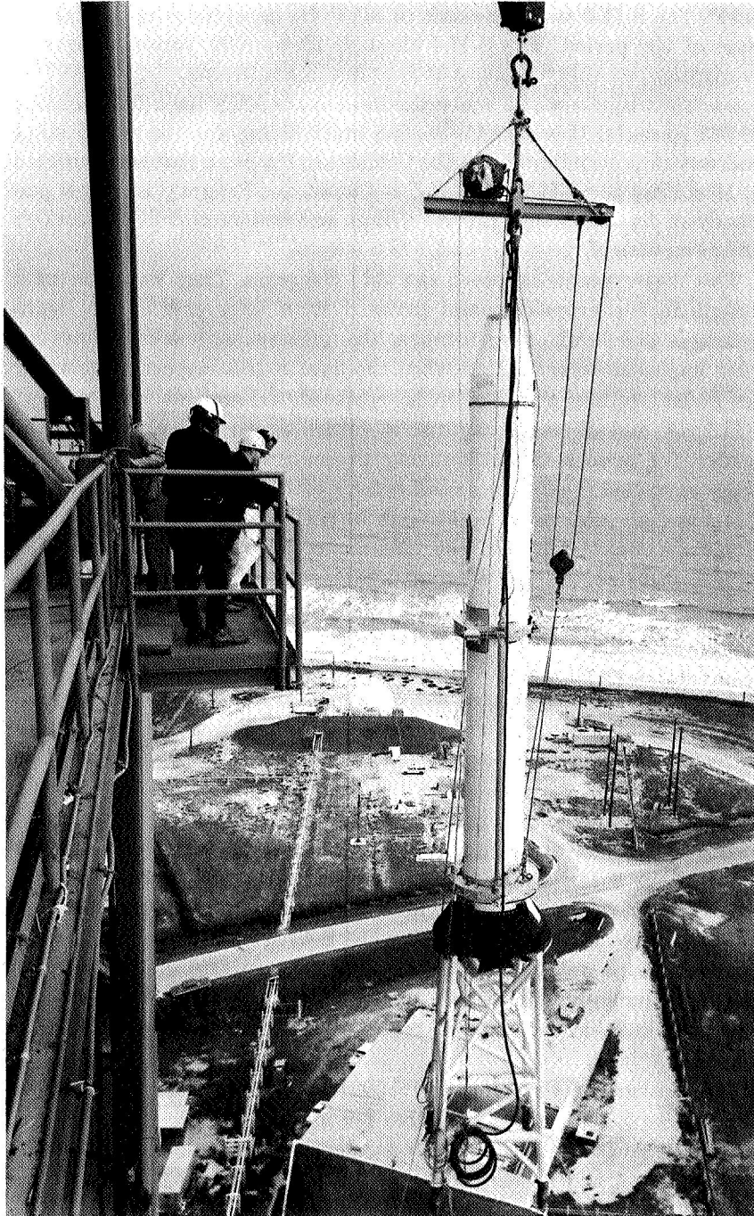
Figure 1-5. Launch Escape System being hoisted to top of service tower.
