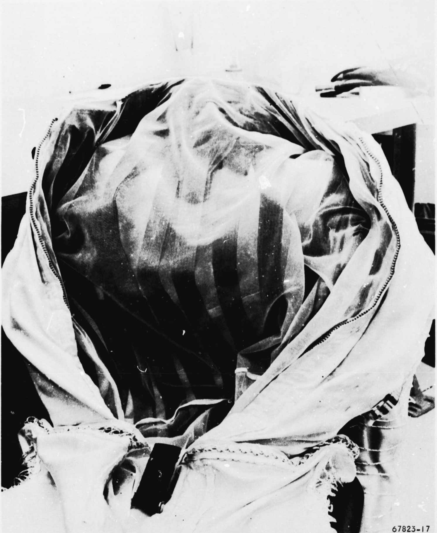
Figure 5. Bladder Suit and Inner Comfort Liner Assembly
