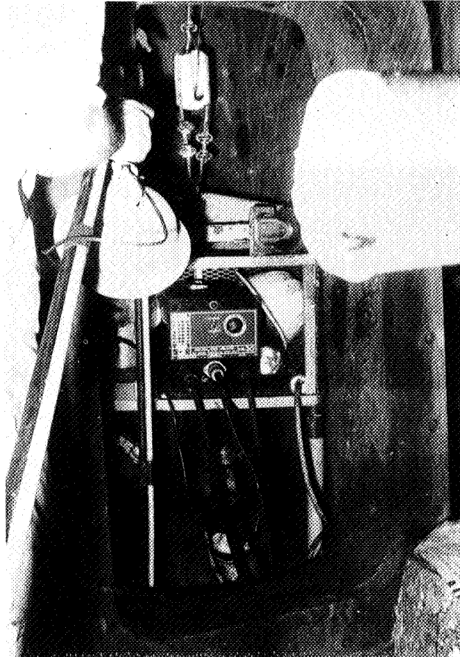
Figure 17.5 Elevator equipment compartment.
