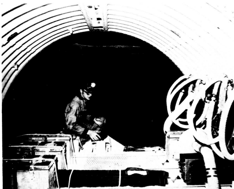
Figure 9.2 Atmospheric conditioning unit.
