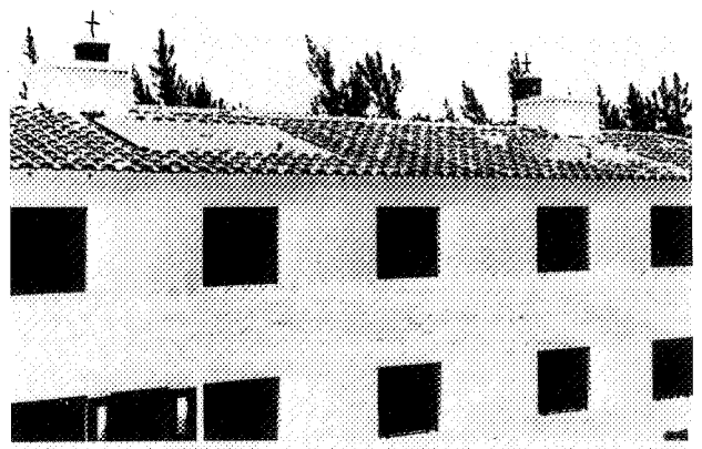
Figure 7. Solar water heaters in an apartment house.
