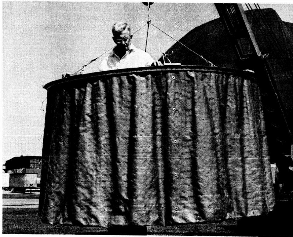
Figure 55. Number 2 Nozzle Extension Assembly
