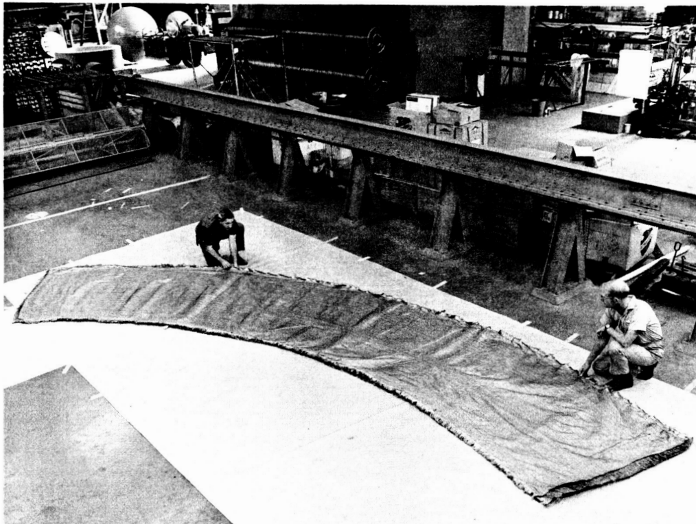
Figure 52. Conical Airmat Woven for Number 1 Nozzle Extension
