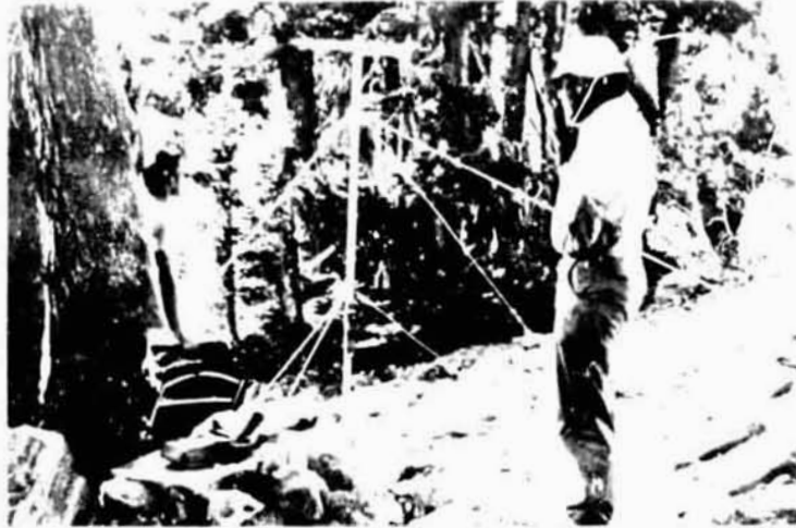
Figure 3: The standard seismic station on Mt. Lassen. The electronics and batteries are in the box in the left foreground. The signal is transmitted in the FM mode to Menlo Park for recording using the VHF antenna shown.
