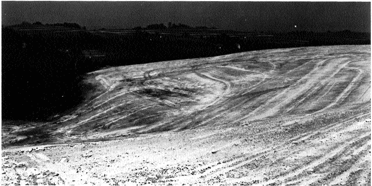
Figure 13. Area reclaimed under terms of the 1972 legislation. Stripped area graded to its original contour prior to planting.
