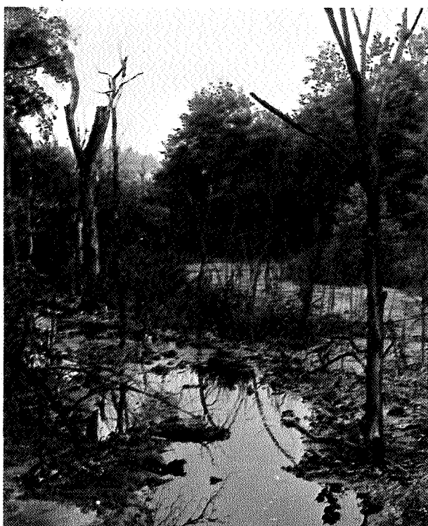
Figure 7. Sediment eroded from spoil banks may fill stream channels, kill vegetation, and cause flooding.
