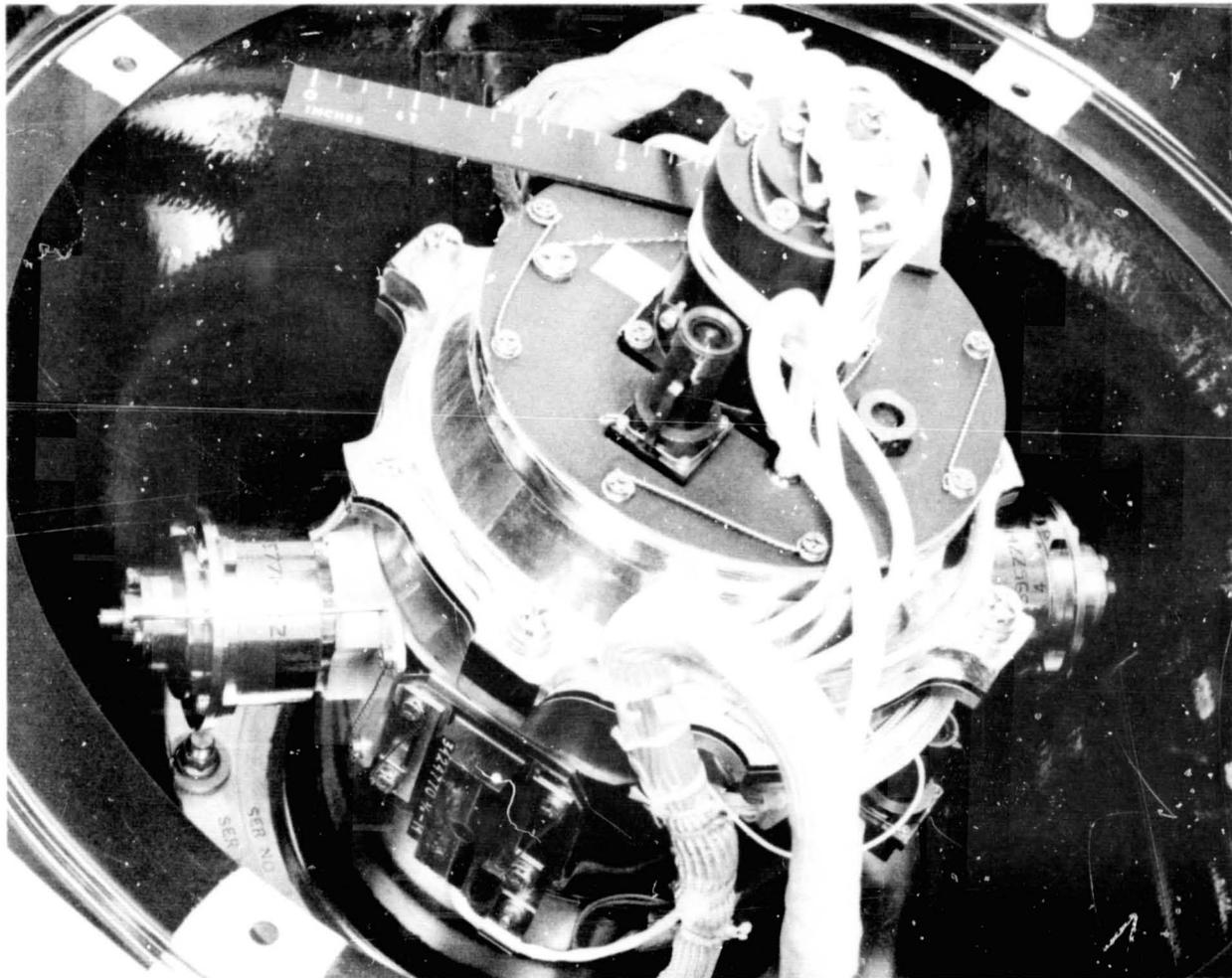
Figure 3. Oiler Installation on IntelSat IVA Despin Assembly
