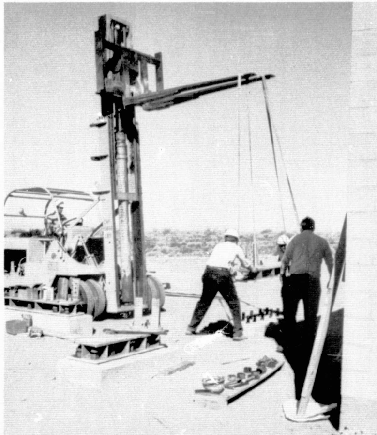
Fig. 27. Radar antenna tower adapter installation
