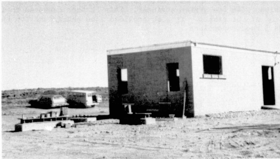
Fig. 26. Partially completed radar site facility
