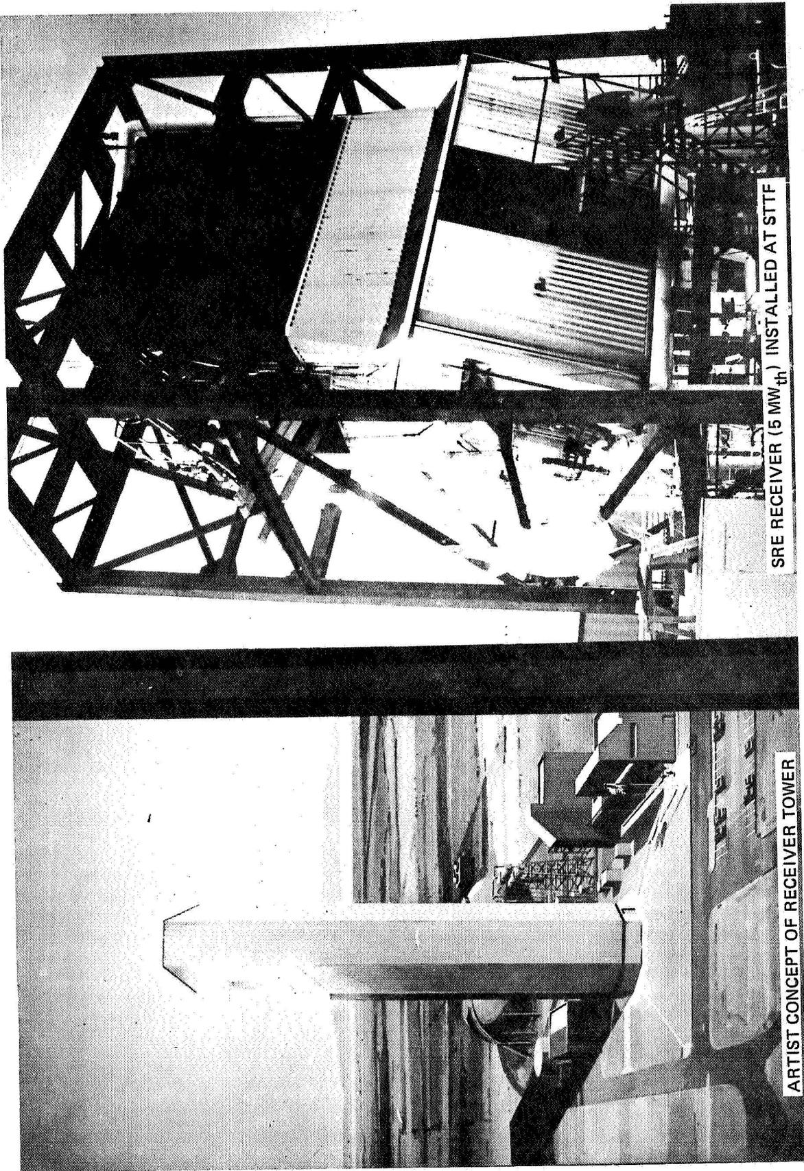
Figure 14. Receiver SRE and tower.
