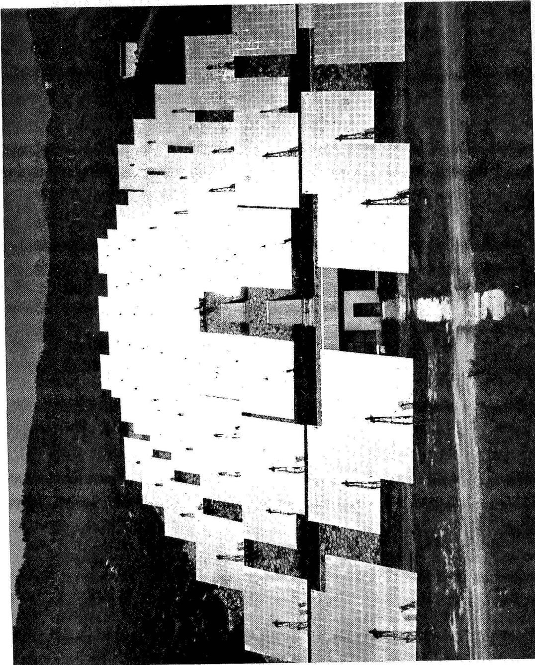
Figure 12. Sixty-three heliostat operation typical of maximum power runs of 1 MW thermal receiver solar test program.
