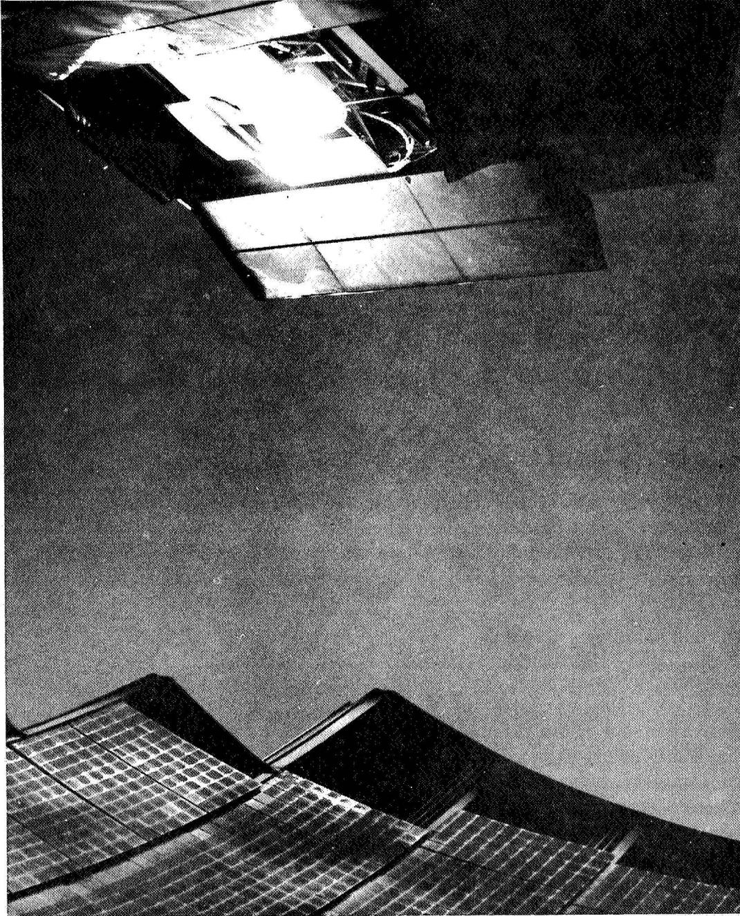
Figure 11. Perspective view of CNRS parabola and focal building with 1 MW thermal cavity receiver in operation — Summer 1976.
