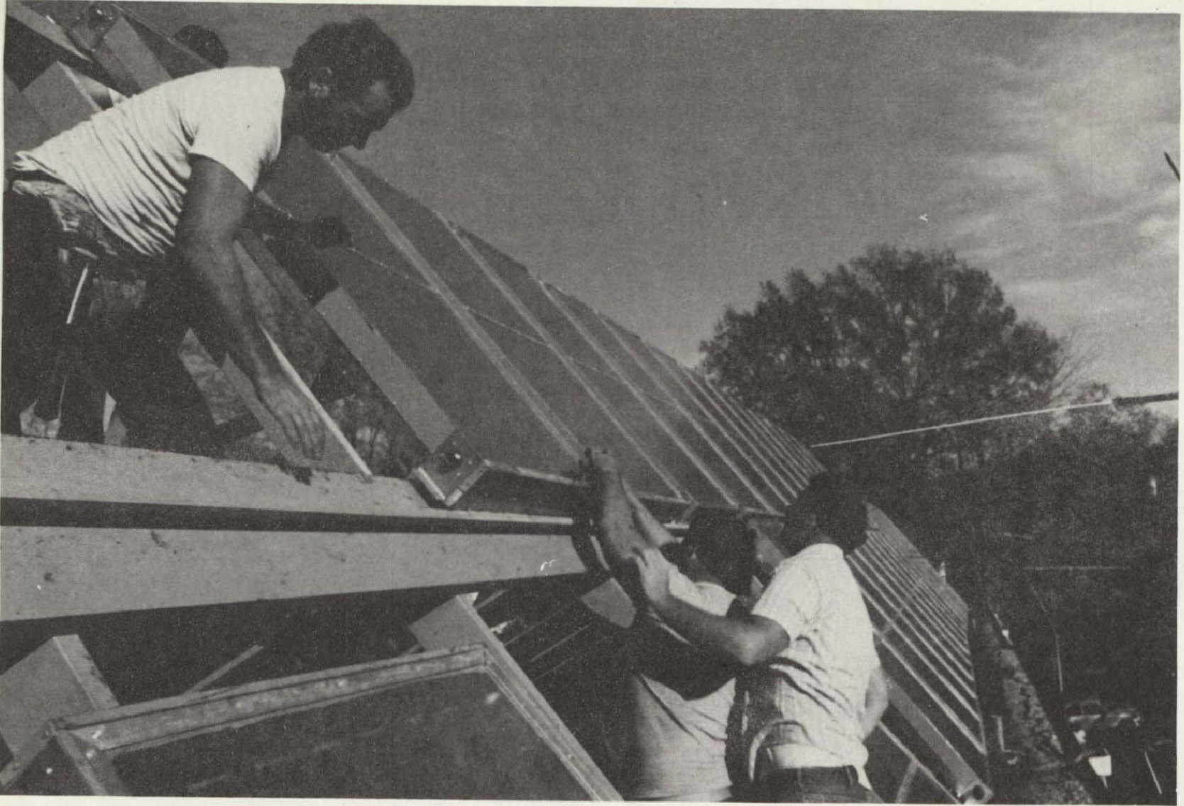
Figure 18. Collector Installation
