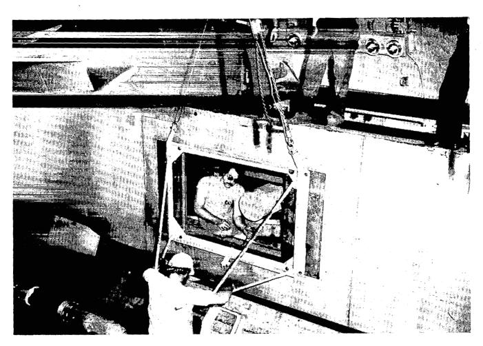
Figure 8.- Installation of tunnel window.
