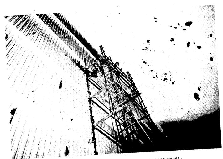
Figure 10.- Installation of bank on turning vanes.
