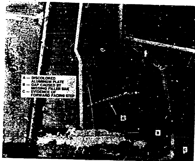
Figure 18.- STS-2 postflight condition of fuselage stub.
