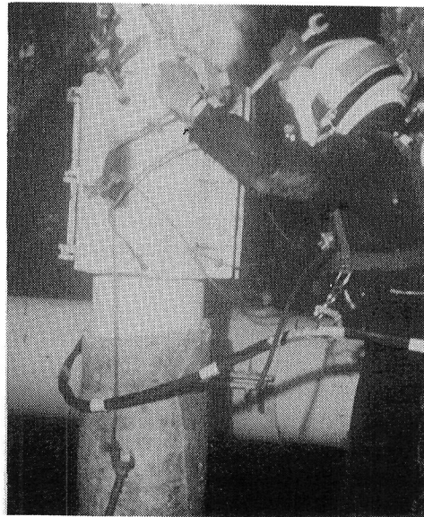
Diver Using an Impact Wrench to Tighten Bolts on a Riser Clamp. Note Use of Legs as Attachment Point
