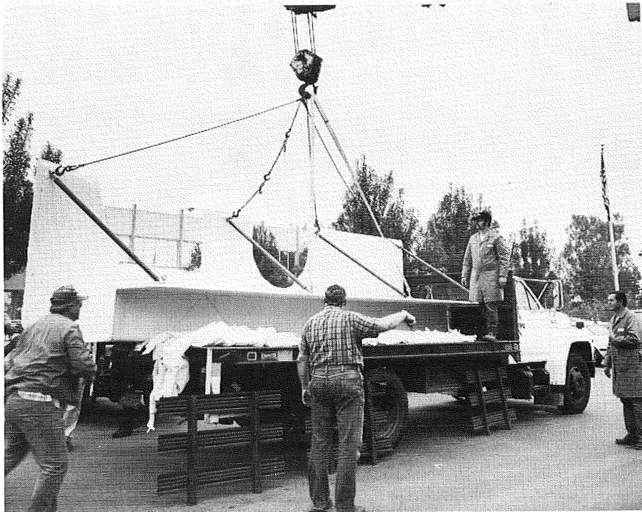
Figure 8. Right Composite Hull Section
