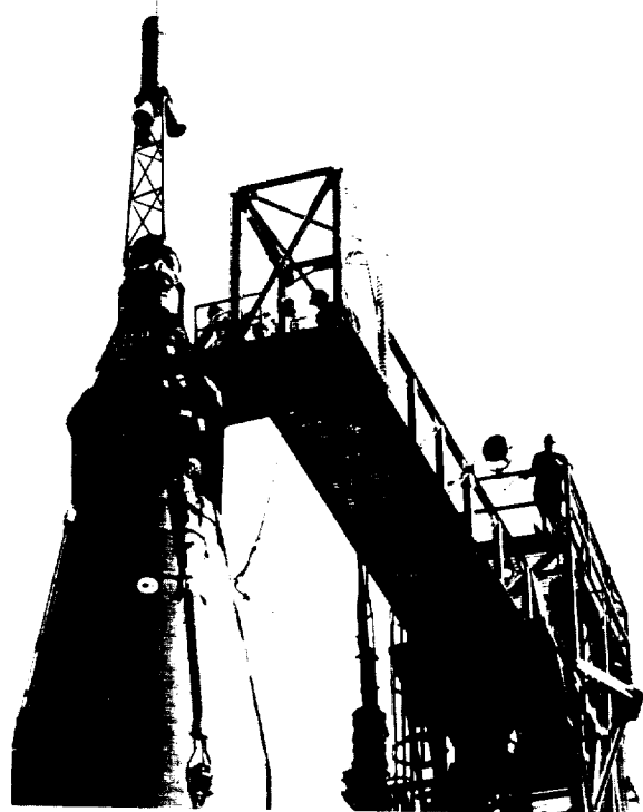
FIGURE 5-24.—Emergency egress tower ramps in place during emergency egress tests.
