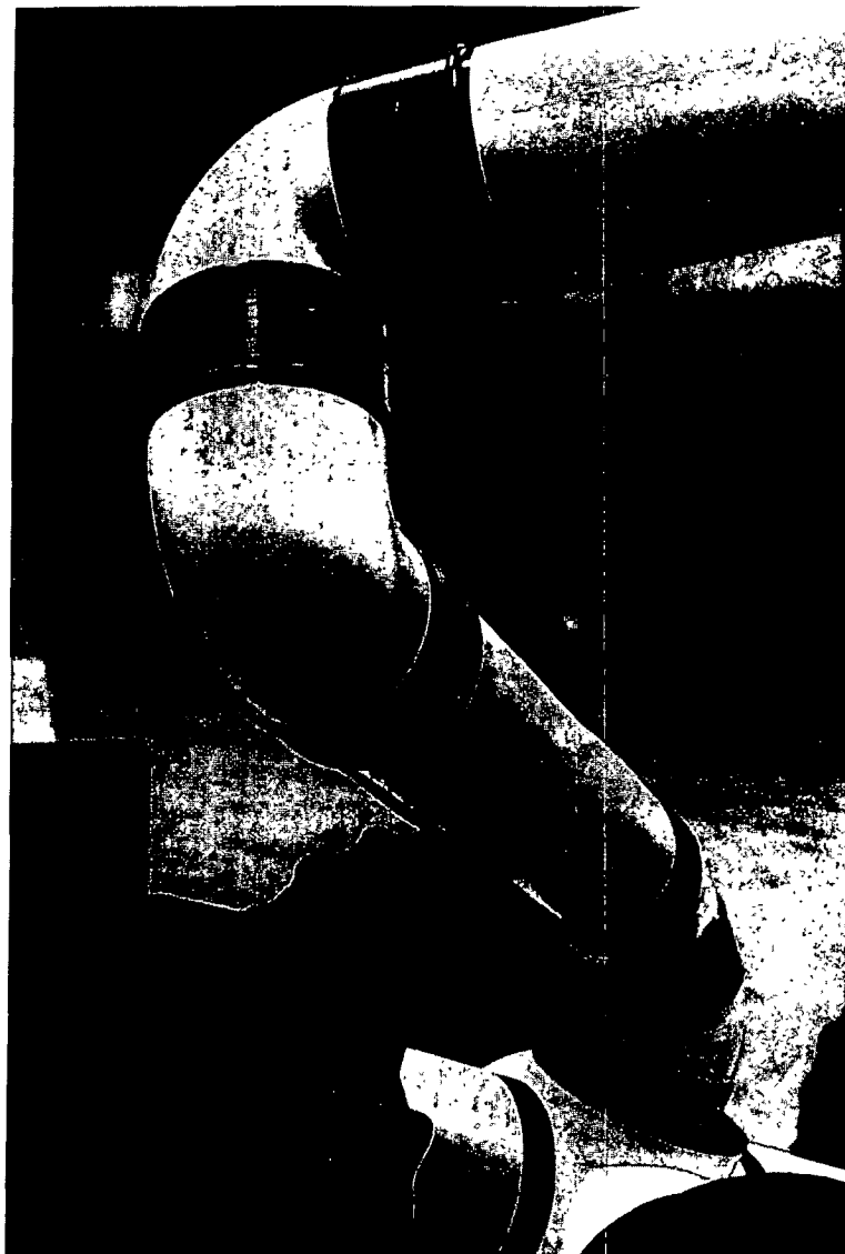
Fig.2 Close-Up View of Articulation Joints
