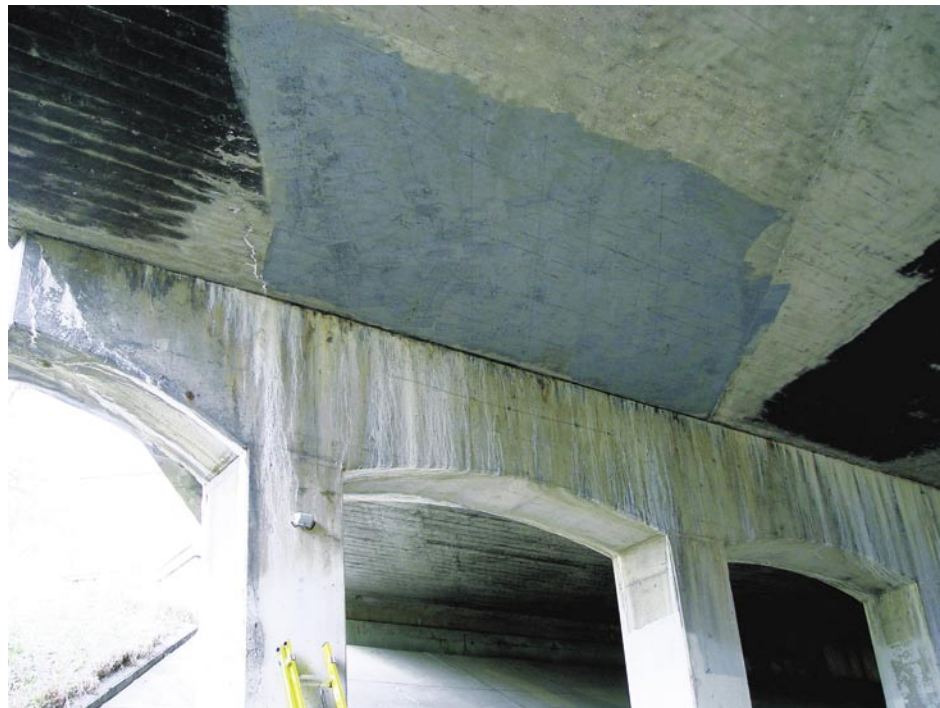
The GalvaCorr™ liquid coating is applied to concrete structures such as this bridge in order to protect the structures from corrosion.
