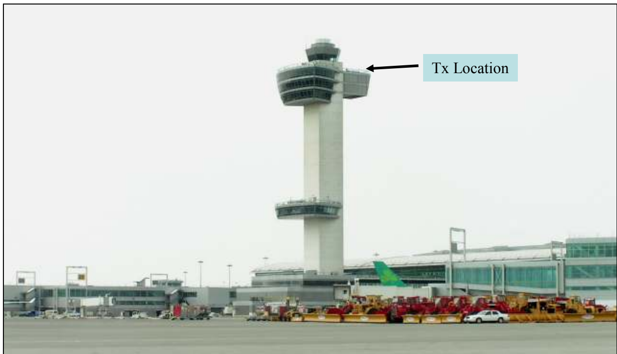
Figure 4.8. Photograph of JFK International Airport ATCT, showing Tx location.
