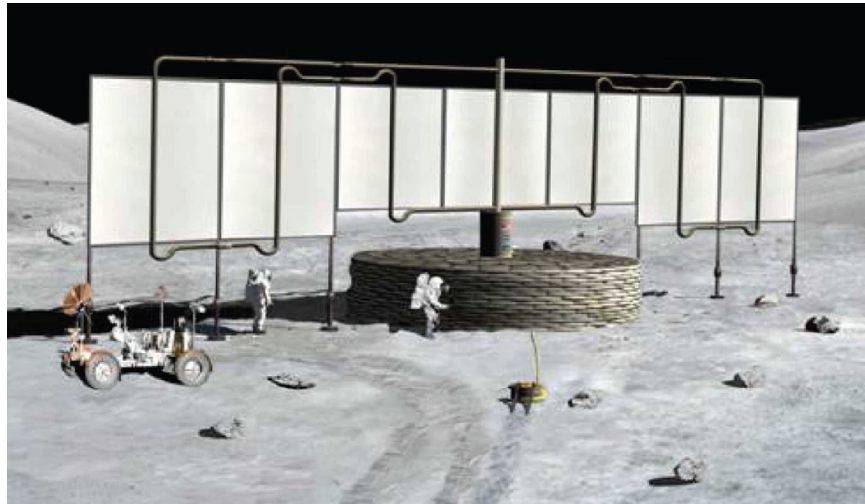
Figure 9.—Fission Surface Power System (FSPS) with regolith sand-bag shielding.
