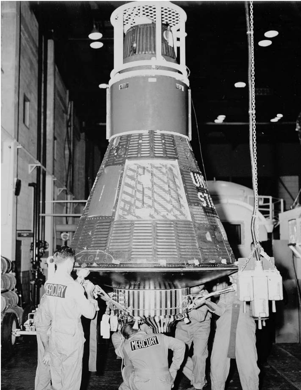
America's first human spacecraft was Mercury. It flew six astronauts into space (two sub-orbital, four orbital) from May 1961 to May 1963. Weighing some 1,360 kilograms (3,000 pounds), the vehicle was launched into space atop the U.S. Army Redstone rocket and later, the Air Force Atlas-D intercontinental ballistic missile. Pictured is Wally Schirra's Mercury 8 capsule Sigma 7 being readied in Hanger S at Cape Canaveral in September 1962. (NASA Image Number GPN-2000-001441)
