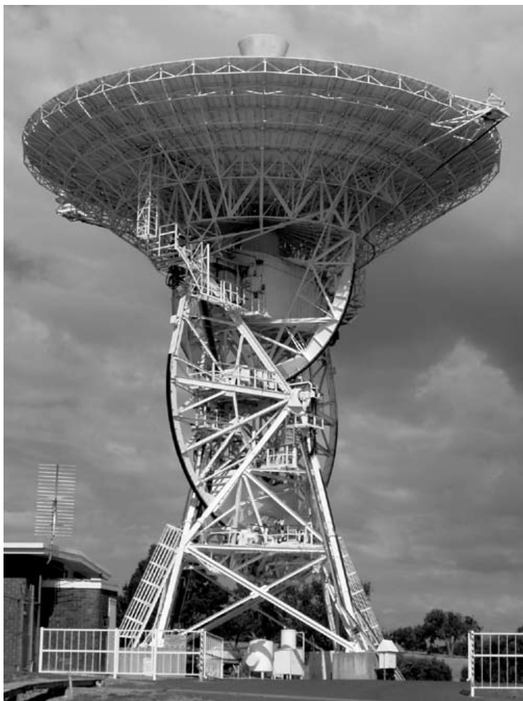
The 85-foot tracking antenna which received signals of mankind's first steps on the Moon on 24 July, 1969 still operates today at the Canberra Deep Space Communication Complex in Tidbinbilla, Australia. The antenna was moved from its original Honeysuckle Creek site some 30 kilometers (20 miles) away in 1985. Clearly visible are the two large yokes which allow the antenna to be moved in two "X-Y" axes as it tracks a spacecraft. (Photograph by the author)
