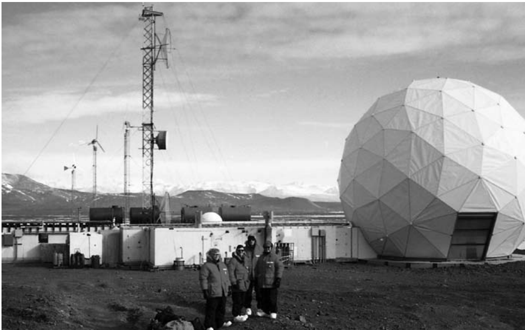
A team from the Goddard Space Flight Center (GSFC) visit the Intelsat communications relay station on Black Island in 1999. Note the microwave tower link back to McMurdo. (Photograph courtesy of NASA)
