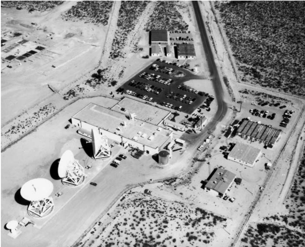
The White Sands Ground Terminal (WSGT) is the central hub of NASA's Tracking and Data Relay Satellite System (TDRSS). It continues the space agency's tracking and data network presence on the south New Mexico Range, a legacy that dates back to 1961. (NASA Image Number HQTC83-907)
