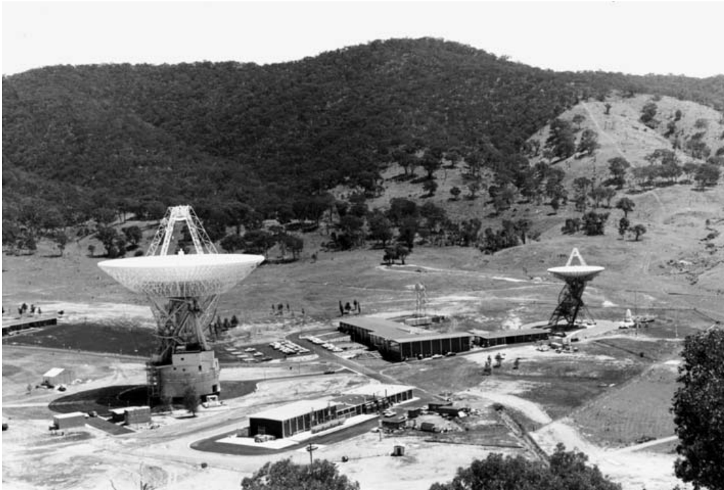
Two 26-meter tracking antennas dominate the skyline of the Rosman STADAN station in the hills of the Pisgah National Forest, North Carolina in this undated photograph. (Unnumbered photograph. Folder 8820, NASA Historical Reference Collection, NASA History Division, NASA Headquarters, Washington DC)
