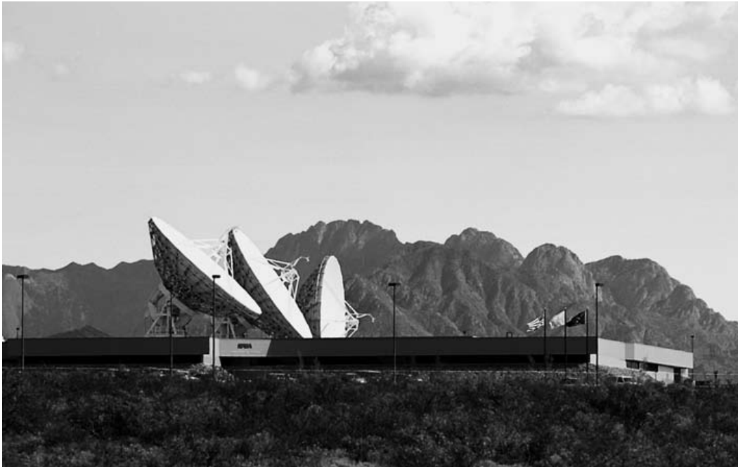
Photograph of the Second TDRSS Ground Terminal (STGT) at the White Sands Missile Range in Southern New Mexico. Towering over the main Operations Building are the three 18.3-meter (60-foot) Ku-band antennas. The San Andres Mountains are in the background. (Photograph courtesy of NASA)
