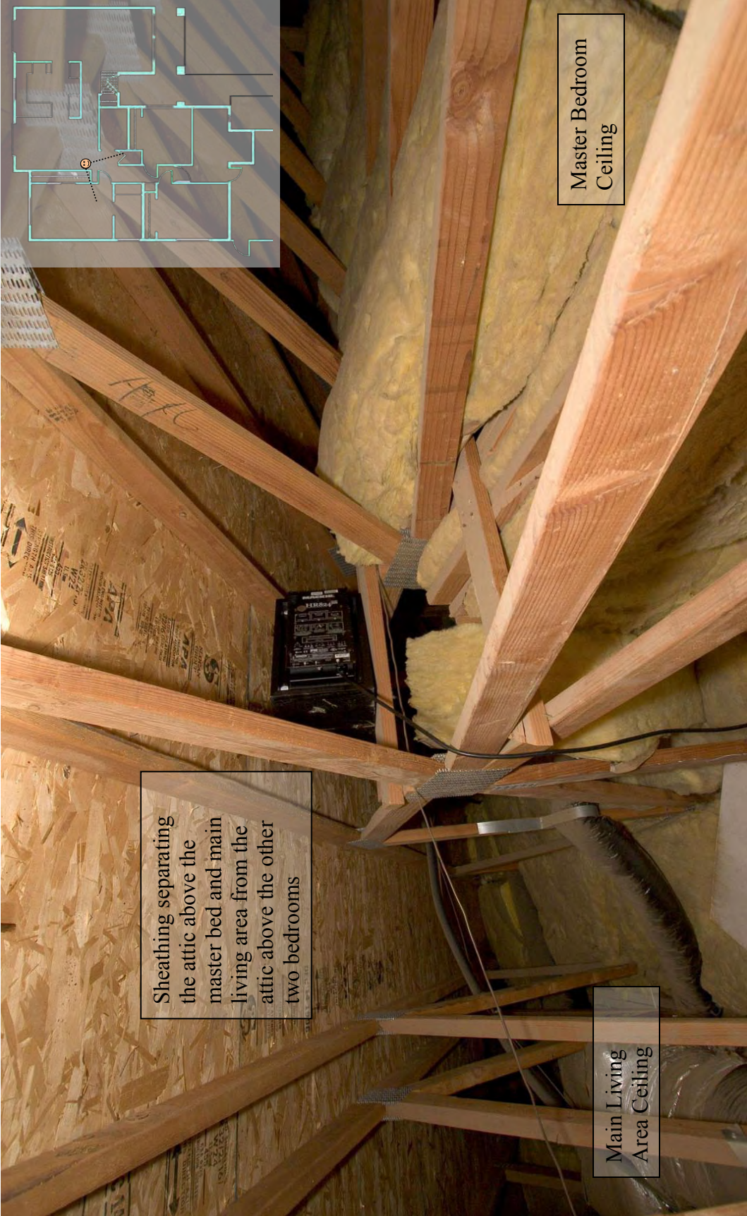
View of the attic above the main living area and master bedroom, looking east, at the sheathing that separates this attic space from the attic above the other two-instrumented rooms. Viewpoint relative to floor plan is illustrated in the inset.
