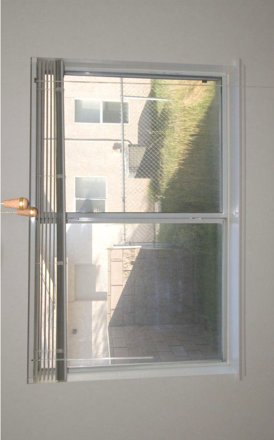
Figure 2.9: Photograph of the window in the garage bedroom. The right side of the window slides open, the left side is fixed.
