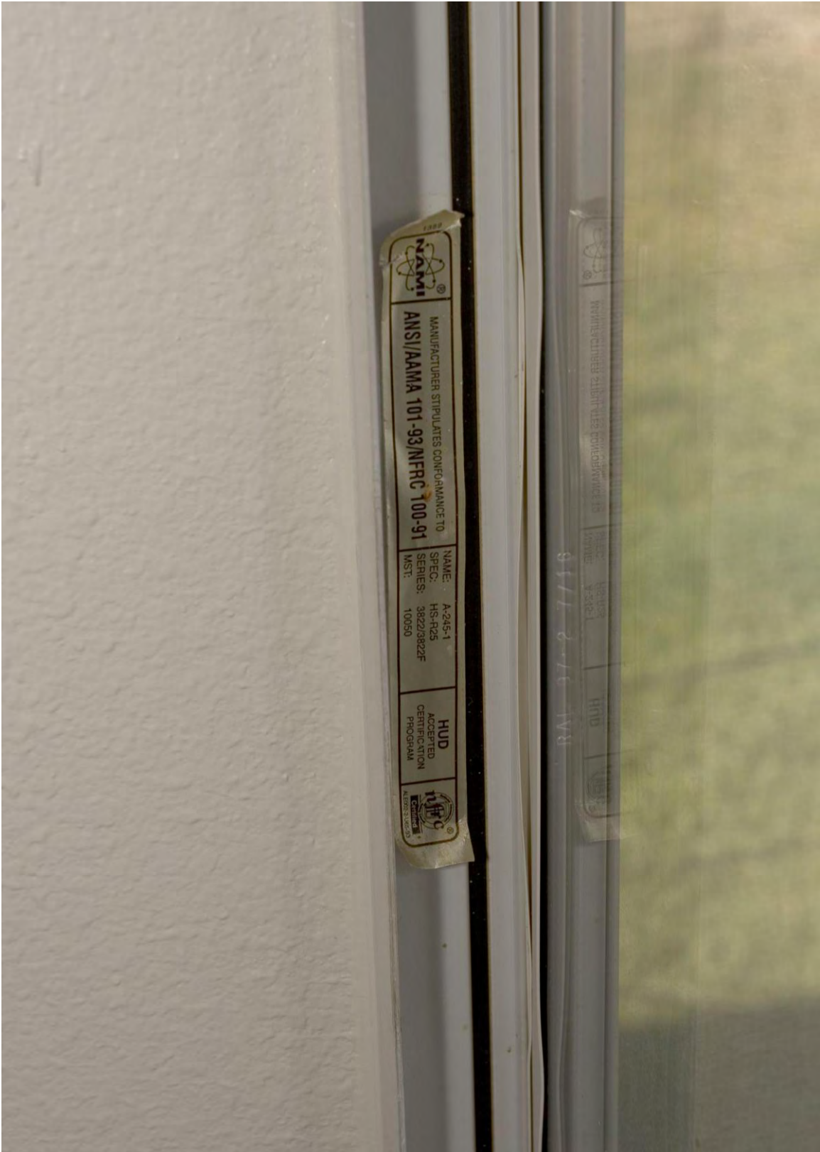
Master bedroom window specification label.
