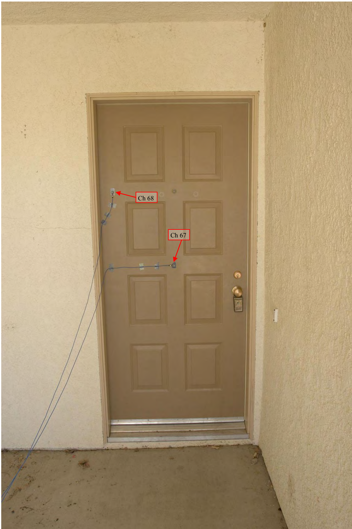
The accelerometers on channels 67 and 68 were removed from the front bedroom and placed on the outside of the front entry door to the house for test on July 18 th 2007.
