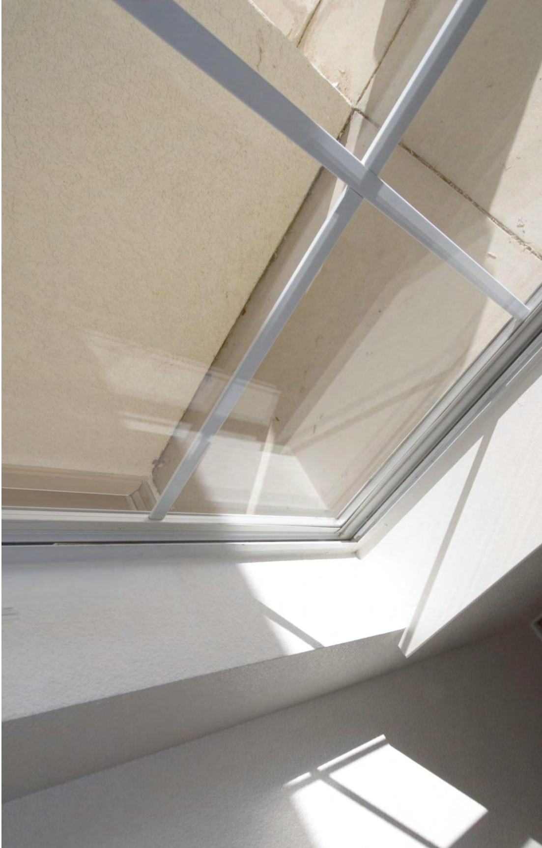
Detailed photograph of the fixed sash of the front bedroom window.
