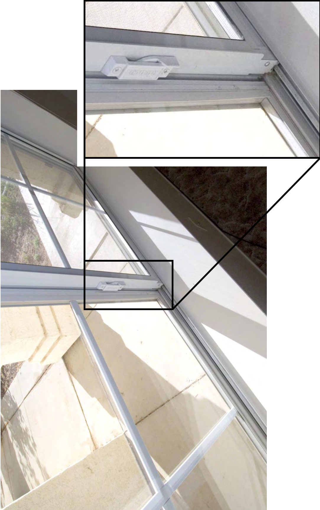
Detailed photograph of both the sliding and fixed sash of the front bedroom window.
