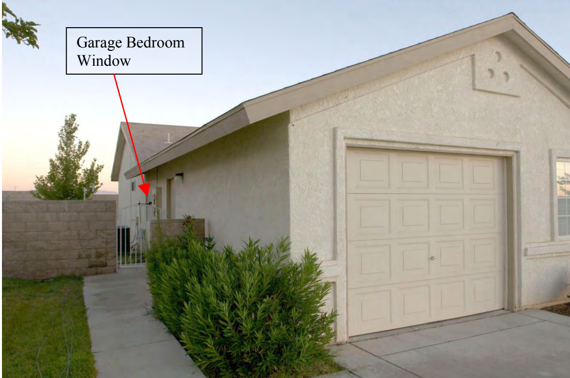
Figure 2.24: View of the side of the house looking northwest at the exterior of the garage.
