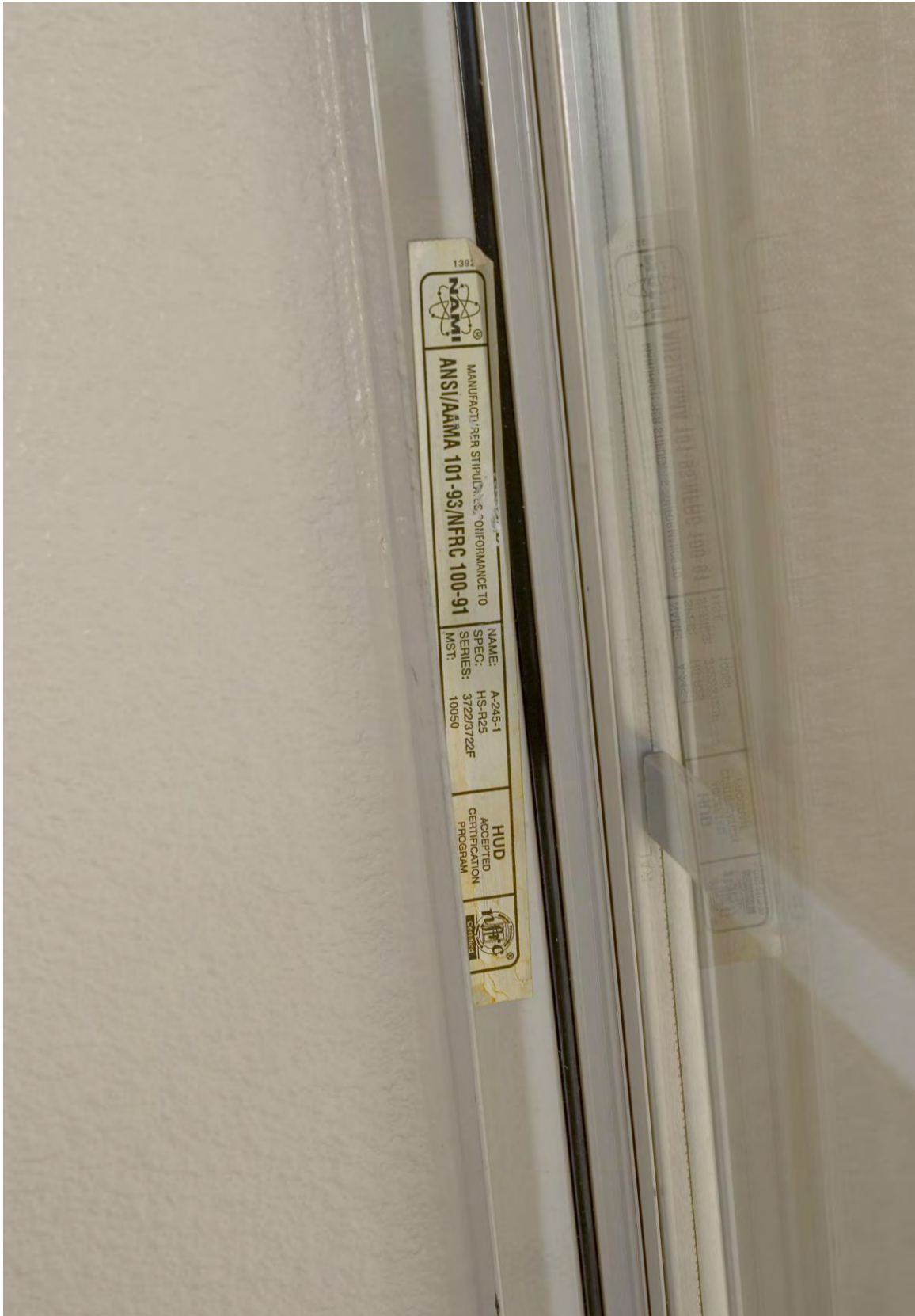
Front bedroom window specification label.
