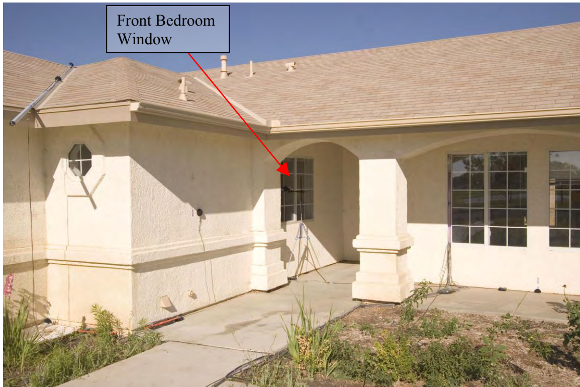
Figure 2.22: View of the front of the house looking south west at the exterior walls of the front bedroom and main living area.
