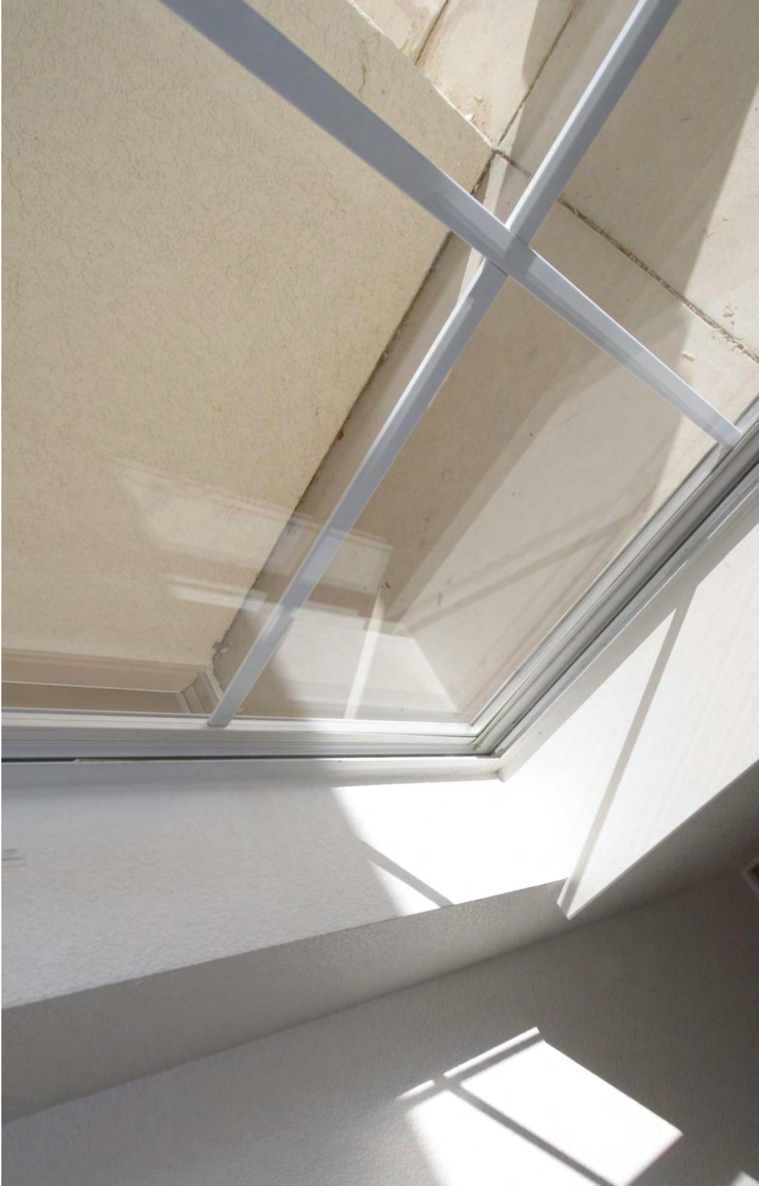
Figure 2.15: Detailed photograph of the fixed portion of the front bedroom window.
