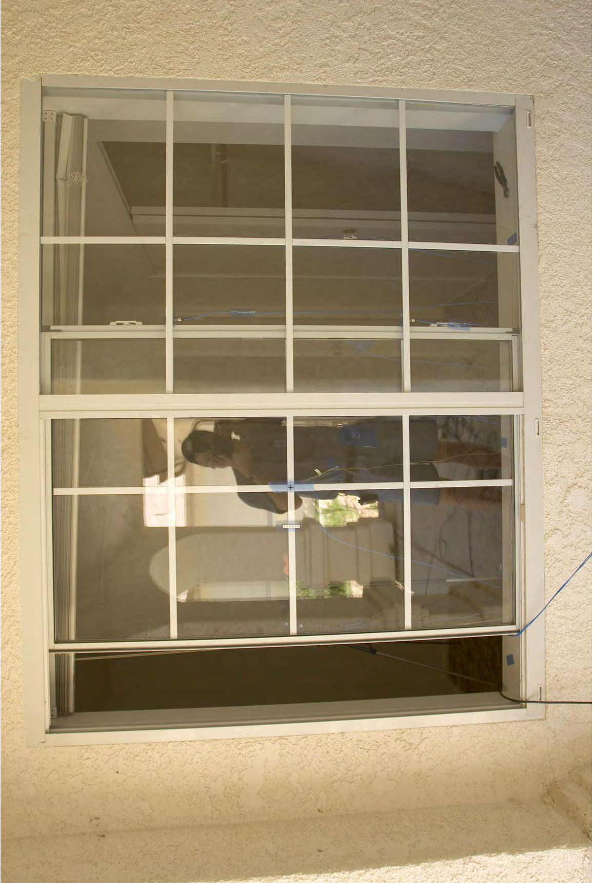
The window for the front bedroom was left cracked open about 6 inches so that the transducer cables could pass to the outside. The window was left open during the boom tests on July 18 th , 2007.
