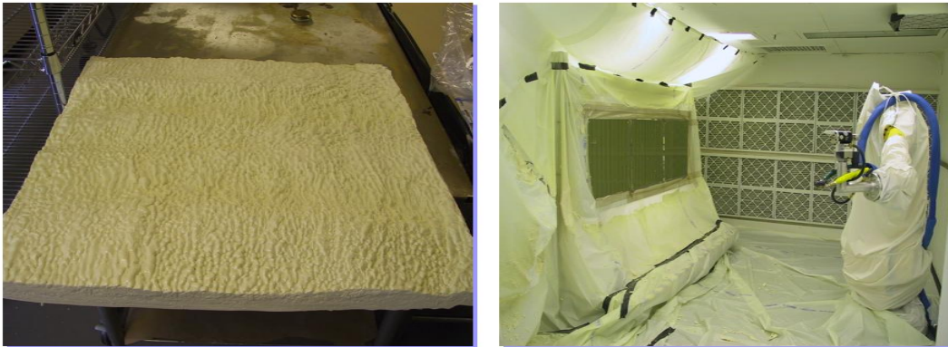
Figure 6. First Upper Stage Foam Panels Sprayed at MSFC.
