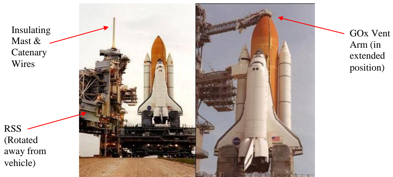
Figure 6.0-1. Pad 39B Lightning Protection
