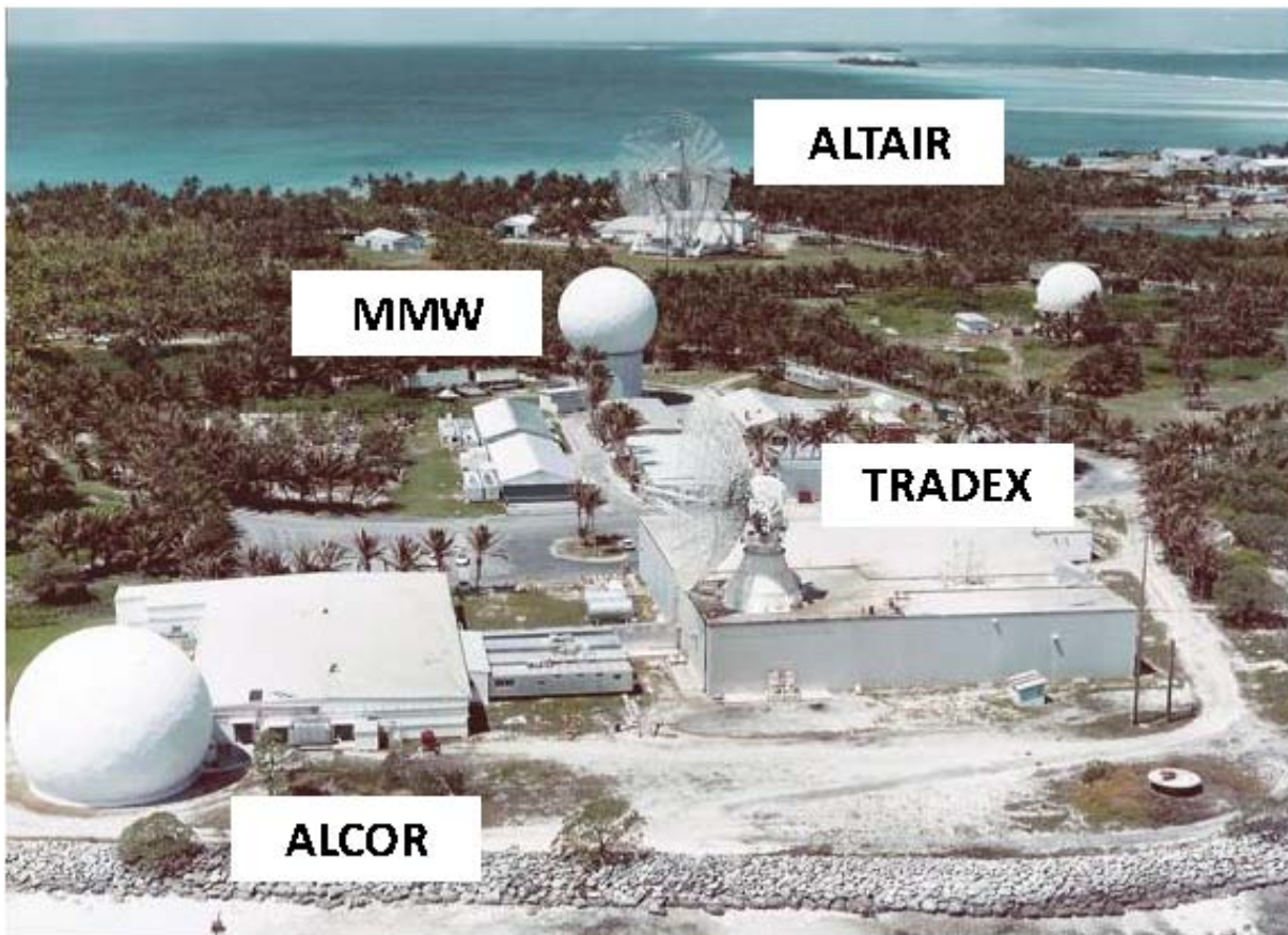
Figure 5. – Four large instrumentation radars located on the island of Roi-Namur, 47 km north of Legan.
