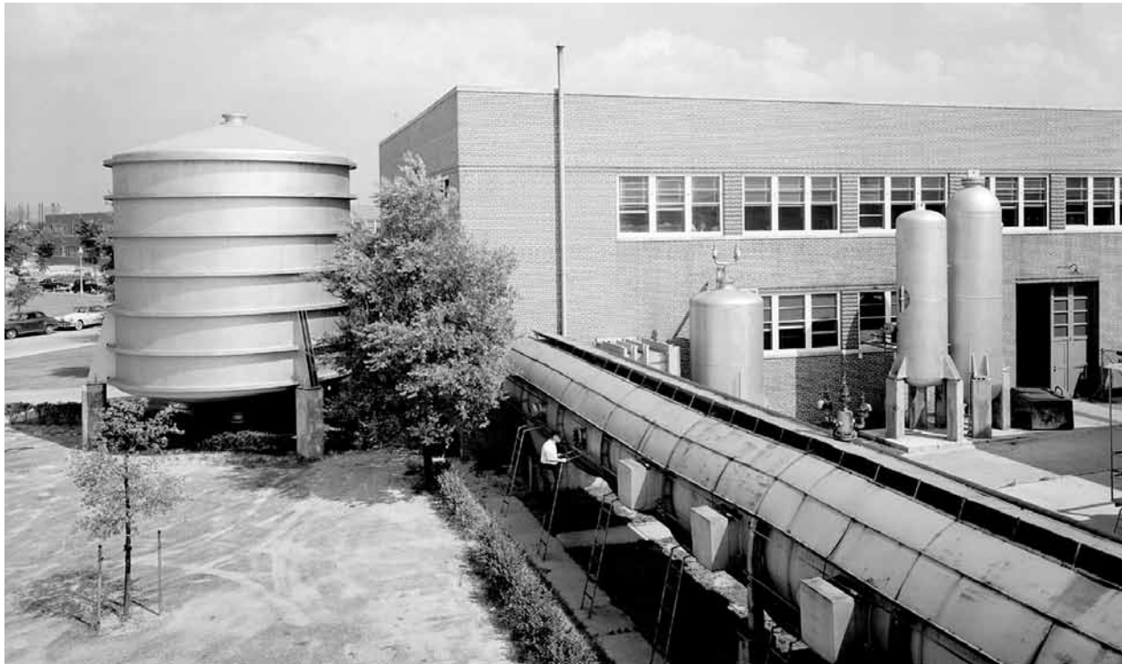
View of the Physical Research Laboratory at Langley in 1949 showing the ill-fated Langley Free-Flight Facility in the foreground. The 100-foot-long, 8-foot-diameter facility was equipped with viewing windows but suffered poor flow characteristics during model flights and was closed before meaningful research results were obtained.
