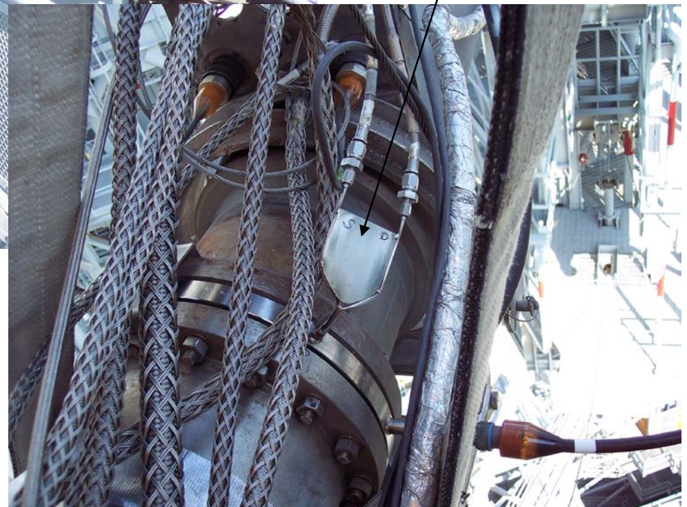
Pitot spool piece installed in Vent line
