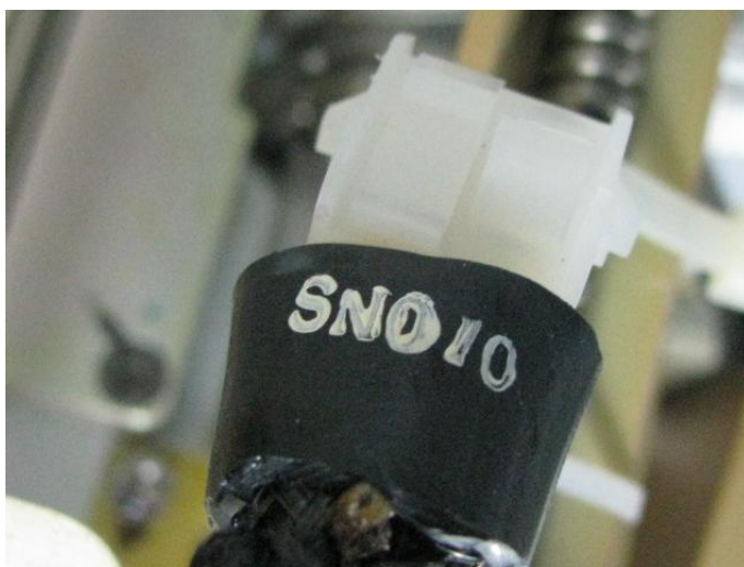
Figure D.12.—Heater 1 Molex connector, note discoloration on wire braid.
