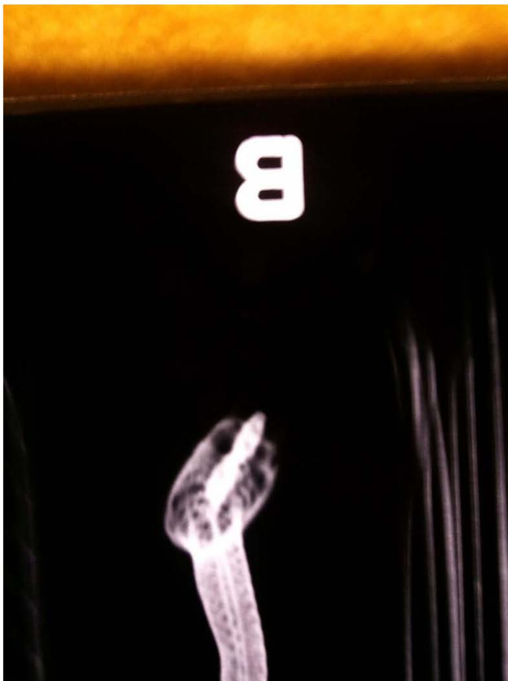
Figure E.89.—Power connection for Bulk Fluid Heater 2.
