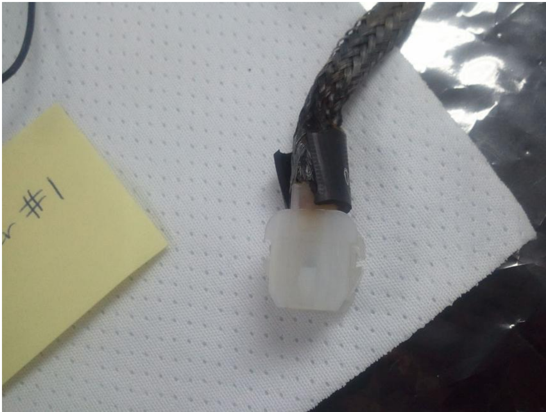
Figure D.47.—Heater 1 Molex connector, note discoloration on wire braid.
