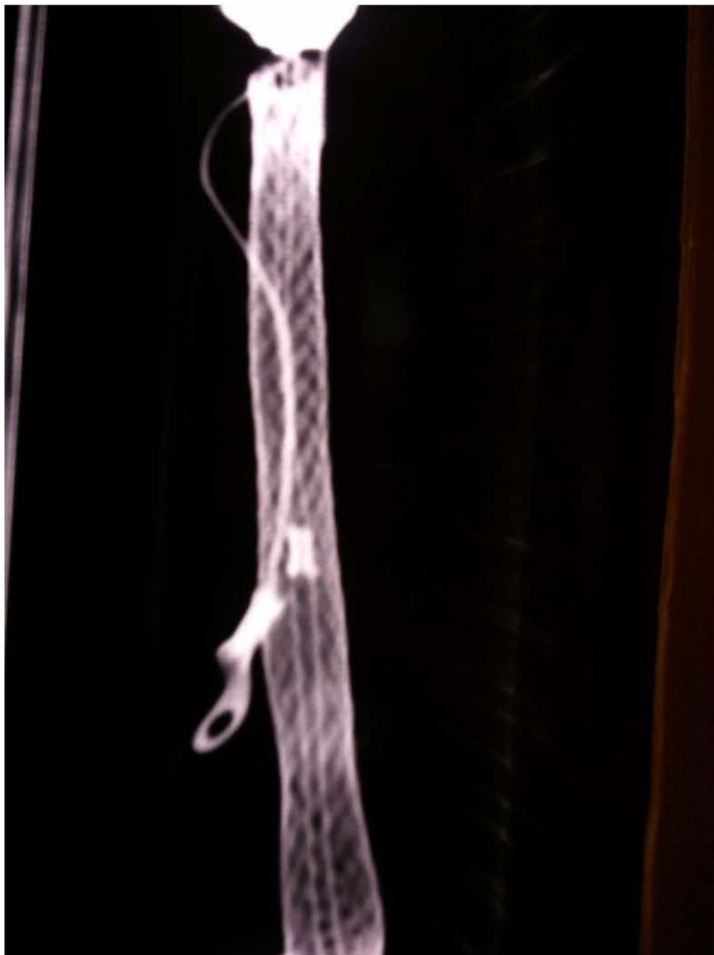
Figure E.86.—Grounding connection for Bulk Fluid Heater 1.
