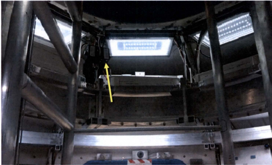
Fig. 7 Custom white LED lighting arrays installed in the plant atrium. Arrow indicates power supply boxes with dimming controls.
