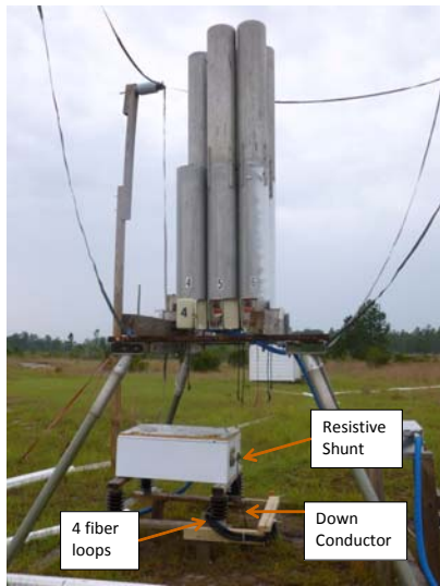
Fig. 13. Four loops of fiber optic current sensor installed under the rocket launch tubes.
