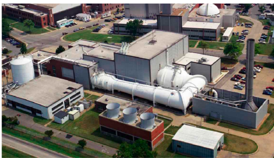
(a) Aerial view of the NTF.
