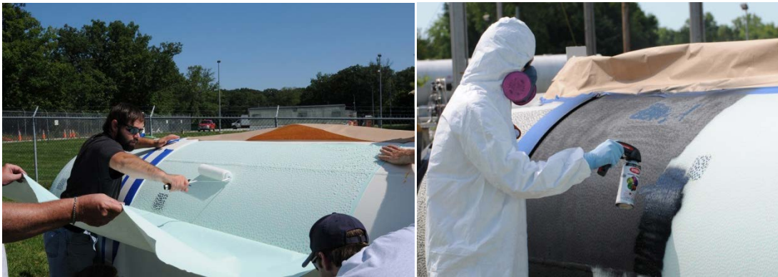
Figure 7.2.3.3-2. Application of Vinyl Stencil (left) and Spray-painting Process (right) on Vessel
