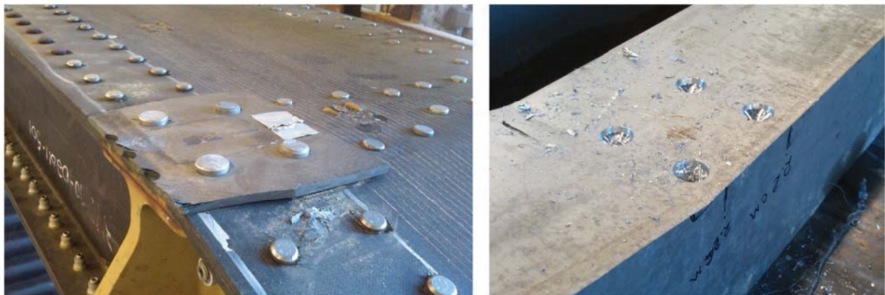
(a) Raised fasteners.
