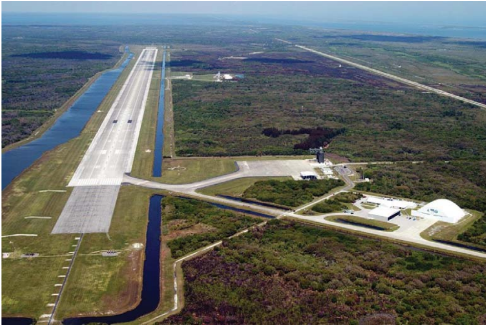
Figure 71. Aerial view of the SLF and associated support structures. Construction has altered 1,350 acres of flatwoods, palm-oak-wax myrtle, palm savanna, and hammocks. An additional 173 acres of fresh to brackish open water habitat was created.
