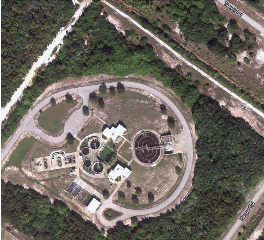
Figure 73. CCAFS waste water treatment facility.
