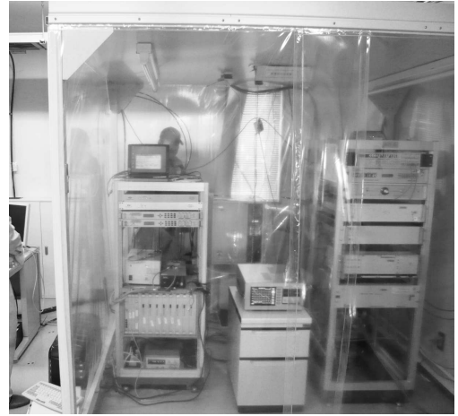
Figure 2. Precise temperature control box located at Kashima 11-m Station.
