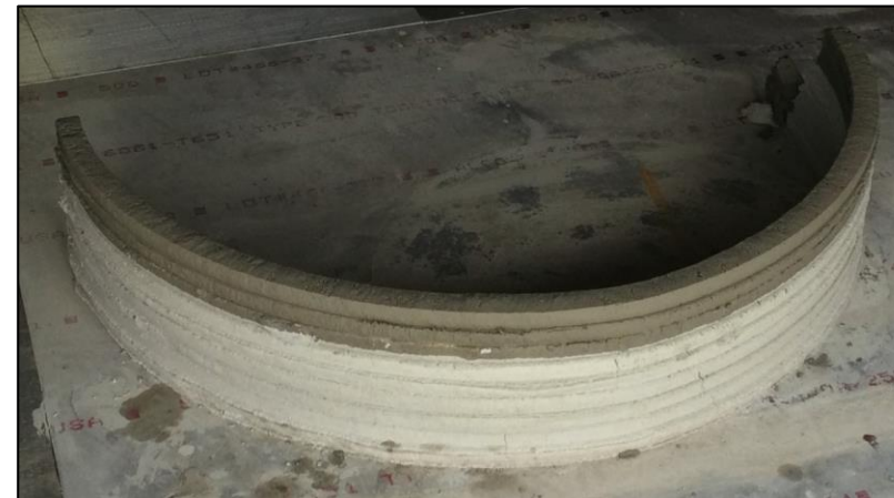
Construction of a curved wall segment using Martian simulant concrete (completed 11/4/15)
