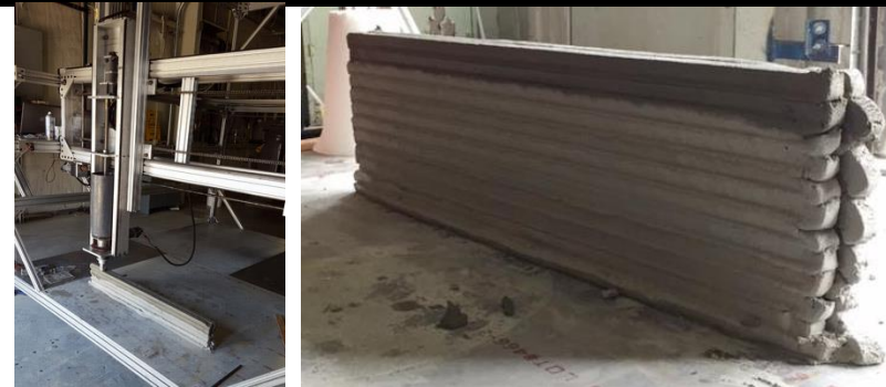
Construction of a straight wall segment using martian simulant concrete, composed of Martian simulant, Portland cement, and stucco mix
