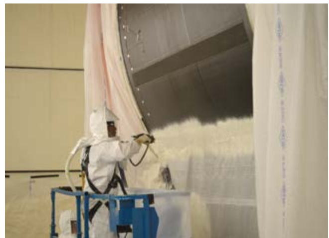
Manual spray foam application to barrel section of the CCTD.
