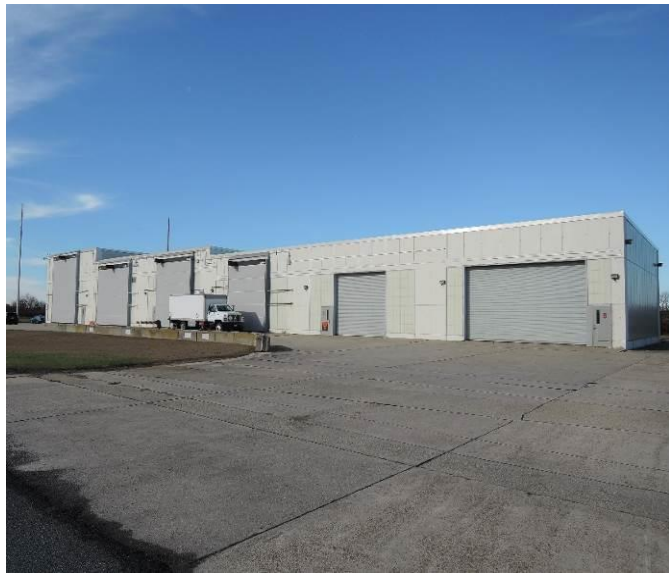
Figure 4: WFF W-65 Facility
