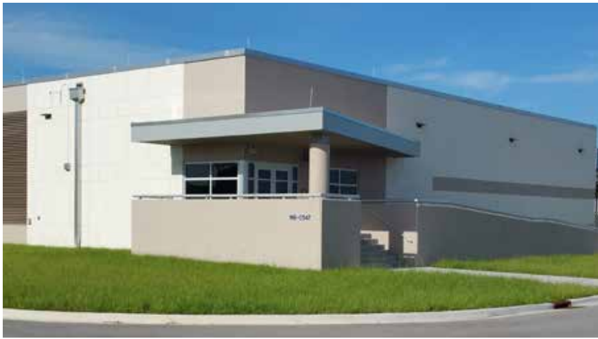
The Data Center Consolidation Project at KSC has successfully migrated three less efficient Data Centers into a new power efficient and more reliable Data Center Facility.
