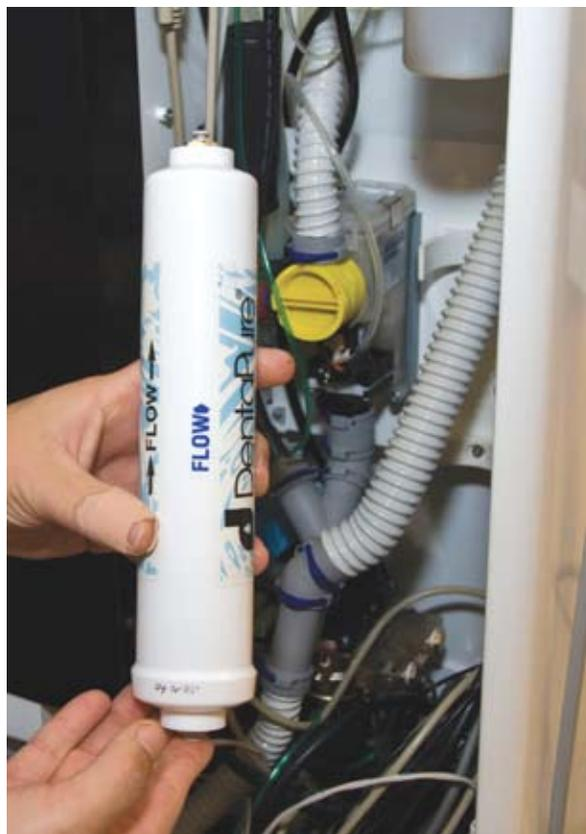
Long service intervals of up to a year and ease of installation make the DentaPure cartridge particularly user-friendly.
