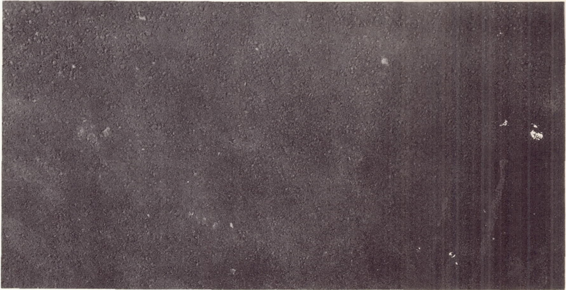
(a) Smooth asphalt runway (sand finish). L-59-7643
