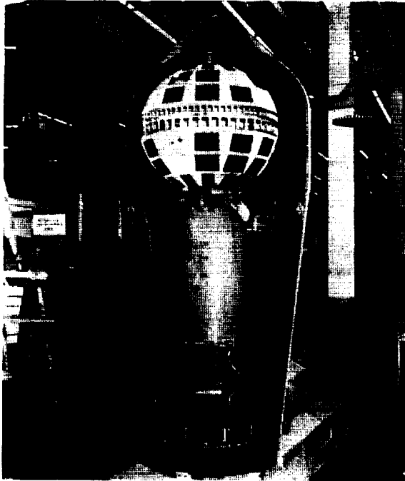
FIGURE 13-5. Telstar test satellite mated to third stage of Delta launch vehicle.
