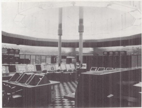
FIGURE 6-17.—Instrumentation controlling servicing, launching, and guiding of vehicle into orbit.
