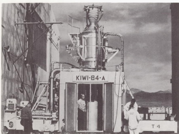
FIGURE 29-3.—Kiwi-B4-A reactor.
