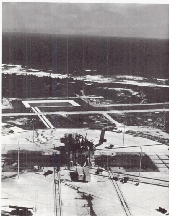
FIGURE 6-19.—Vertical Launch Pad 34.
