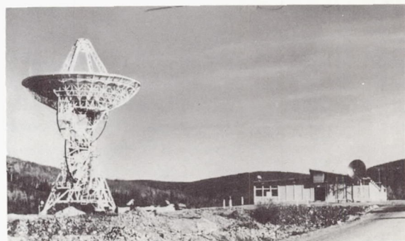
FIGURE 9-15.—Command and Data Acquisition Station, Fairbanks, Alaska.
