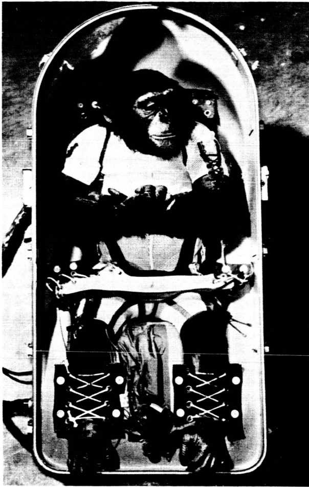
FIGURE 3-2.—Animal in couch (compare with fig. 2-2). The lacing on the arms to fit the adjustable nylon restraint suit is visible. The waist panel with its zipper which is attached to the couch lid can also be seen.
