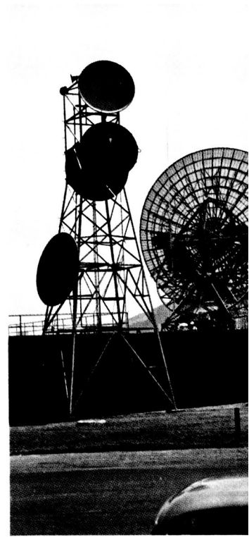
Data gathered at Goldstone are transmitted to the SFOF at JPL by teletype and high-speed digital data circuits over a microwave link.
