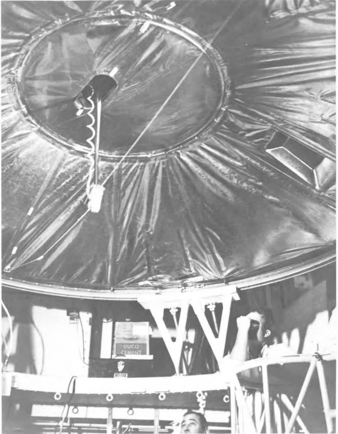
Figure 12-4.- Magnetometer boom extension.
