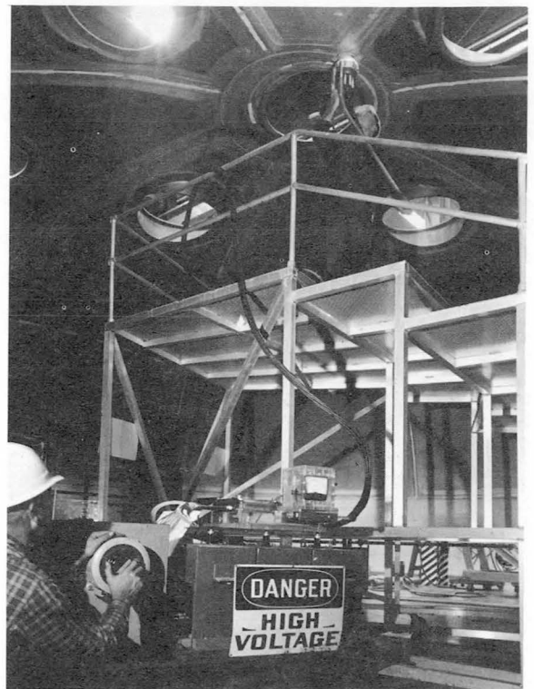
FIGURE 23.—Distortion removal from finished Saturn bulkhead, or tank end.
