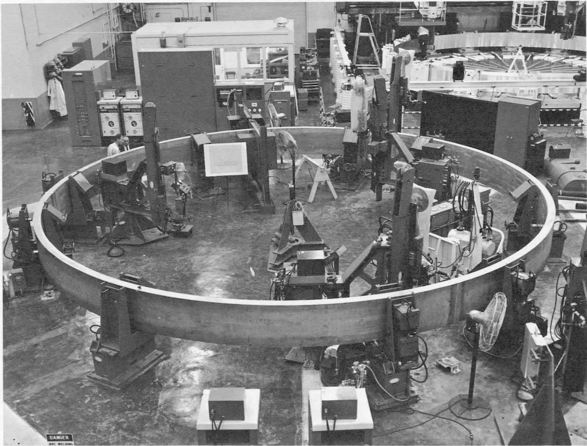
FIGURE 11.—Welded 2219 aluminum alloy Y-ring billet prior to machining.
