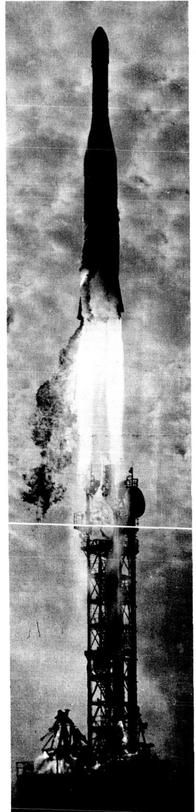
the sustainer engine was shut down and the velocity properly adjusted with two small rocket engines. Then the huge, empty Atlas was detached and Agena took over. Before the Agena engine was started, the aerodynamic nose cover had to be jettisoned. This time, it came off easily.
